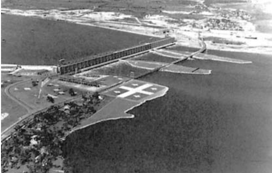
Figure 9 The Beauharnois generating station on the St. Lawrence River contains 26 3-phase alternators rated 50 MVA, 13.2 kV, 75 r/min, 60 Hz at a power factor of 0.8 lagging. An additional 10 units rated 65 MVA, 95.7 r/min make up the complete installation. The output ranges between 1000 MW and 1575 MW depending upon the seasonal water flow. (Courtesy of Hydro-Québec)
