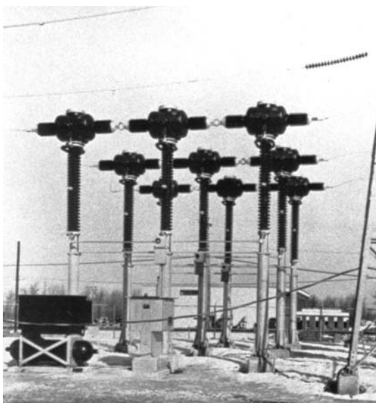
Figure 5 Air-blast circuit breaker rated 2000 A at 362 kV. It can interrupt a current of 40 kA in 3 cycles on a 60 Hz system. It consists of 3 identical modules connected in series, each rated for a nominal voltage of 121 kV. The compressed-air reservoir can be seen at the left. Other characteristics: height: 5640 mm; overall length: 9150 mm; BIL 1300 kV. (Courtesy of General Electric)
