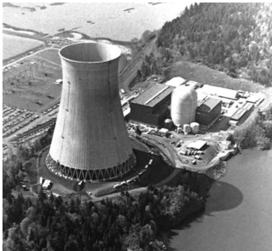
Figure 21 Cooling tower installed in a nuclear power station in Oregon. The generator output is a 1280 MVA at a power factor of 0.88. Tower characteristics: height: 152 m; diameter at the base: 117 m; diameter at the top: 76 m; cooling water: 27 m 3 /s; water loss by evaporation: 0.7 m 3 /s. The temperature of the cooling water drops from 44.5° to 24° as it passes through the tower. (Courtesy of Portland General Electric Company)
