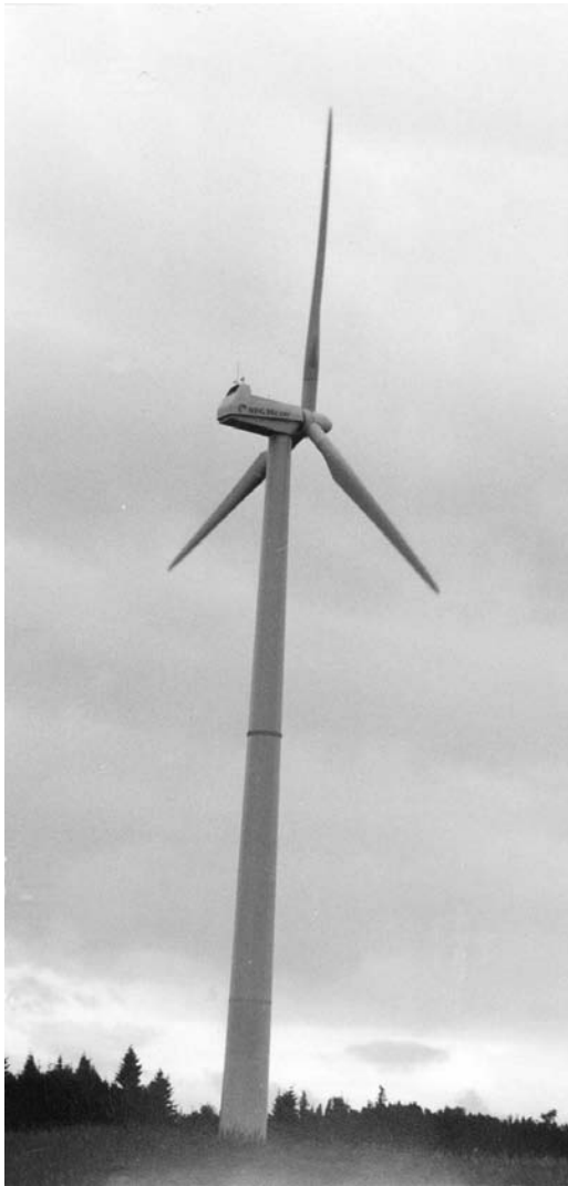
Figure 38b The nacelle (also called pod) is set on top of a 55 m steel tower. The pod is 8.5 m long and it automatically yaws to face the wind at all times. It is equipped with a lightning arrester and is heated during the winter.
