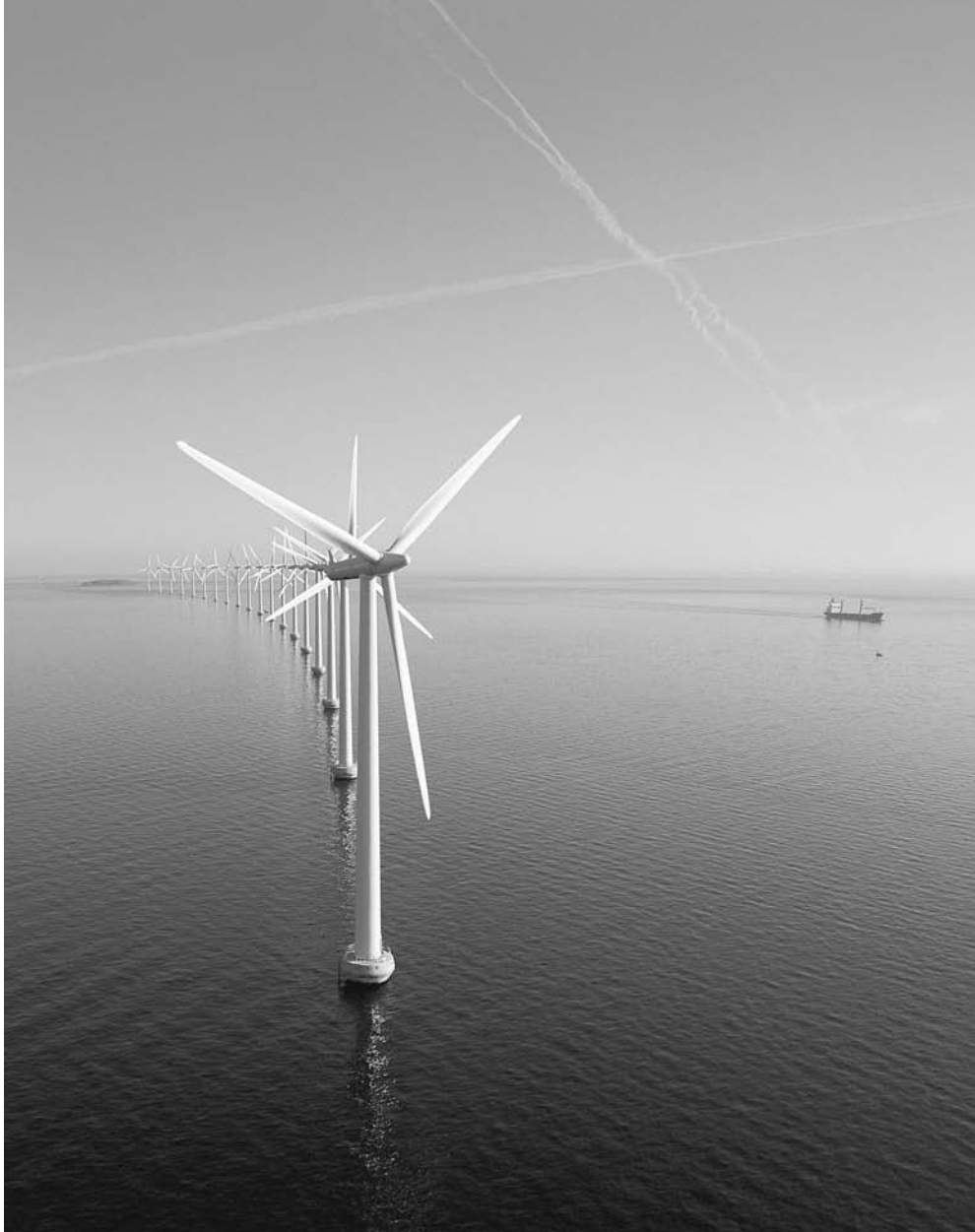
* This Middelgrunden Offshore Wind Farm is located just outside Copenhagen Harbour, in Denmark. It consists of twenty 2 MW turbines yielding a total output of 40 MW. The blades are 38 m long, revolving at a hub height of 64 m. The twenty turbines are equipped with squirrel-cage induction generators that together produce a guaranteed minimum of 89 000 MW h per year. (Photo © BONUS Energy A/S)
