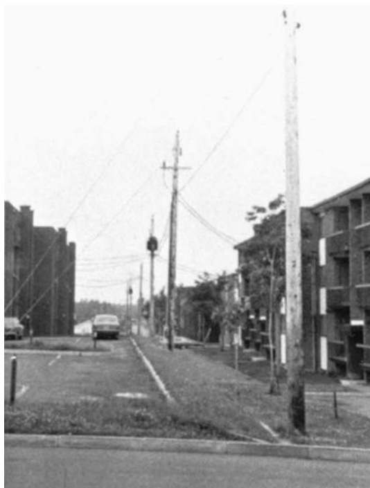
Figure 28 MV aerial feeder serving a residential district.
