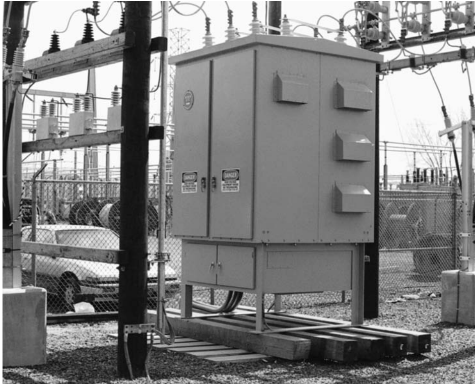
Figure 33 This 13.8 kV, 3-phase solid-state circuit breaker (SSB) comprises both GTOs and thyristors. The GTOs are rated 600 A and the thyristors are rated for 8000 A. (Courtesy of Westinghouse Electric Corporation)
